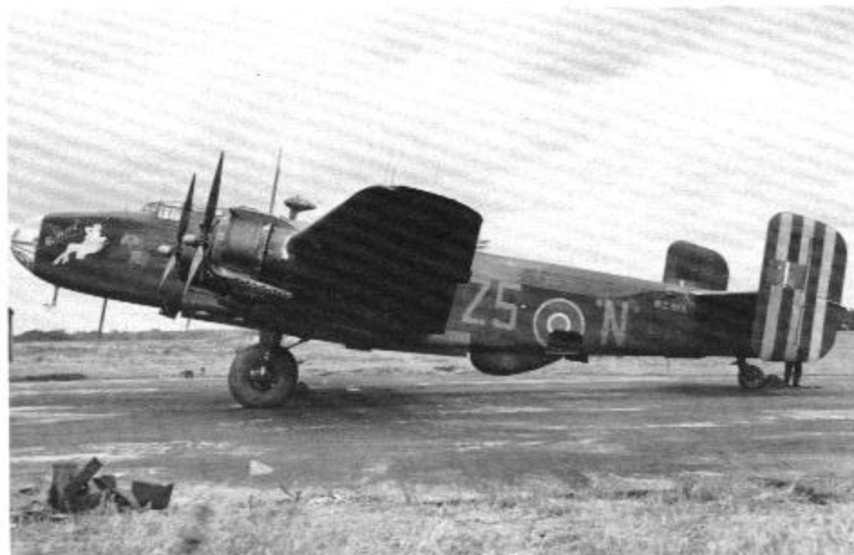
No 462 (RAAF) Squadron Halifax B III with full 'Airborne Cigar' fit for radar-jamming duties. Of additional interest are the wing-tip 'Pipe Rack' jammer whip aerials, the 'Window' chutes forward of the bomb doors and aft of the H2S cupola and the bulged fairings on the inner sections of the bomb doors. 'Jane' also carries No 4 Group daylight identification markings of three yellow vertical tail stripes, even though it was part of No 100 (BS) Group from January of 1945. (M. Wright)
