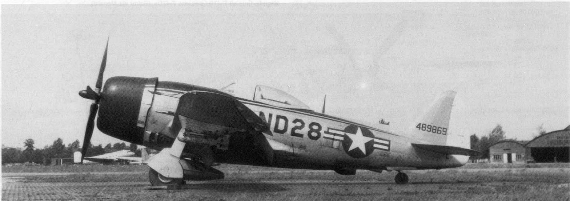
(Below) A F-47D-35 from the 527th FSq/86th FGp on the ramp at Munich in March 1949. The D-35 had four rocket launch stubs under each wing. The entire cowl and stripe under the antiglare panel is Red, while the rudder is White. (Olmsted)
