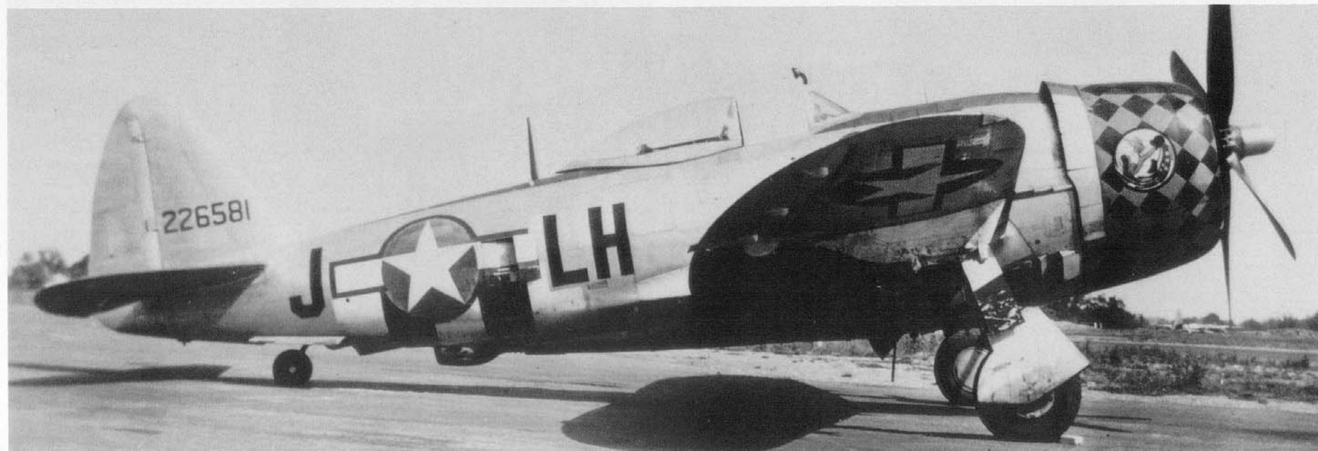
(Below) A P-47D-25 from the 350th FSq/353rd FGp. The extreme bulk of the Thunderbolt is evident in this photo. The nose checks are Black and Yellow. Note the New Blue surround to the national insignia and D-Day stripes on the underside of the aircraft only. (AFM)
