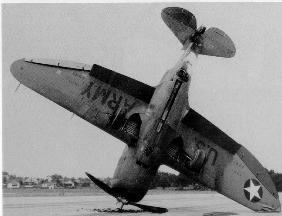
(Below) A P-43A from the 122nd Reconnaissance Squadron, Louisiana National Guard, that ground looped at Winston-Salem in 1942. The turbosupercharger installation can be seen running along the belly. (AFM)
