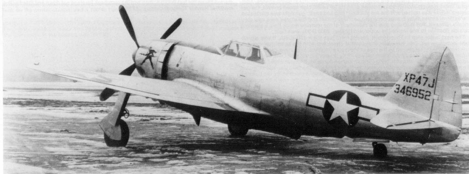
(Below) The XP-47J was the fastest Thunderbolt to fly. It was powered by a 2800 hp R-2800-57 in a lightened airframe and achieved 505 mph on 5 August 1944. (AFM)
