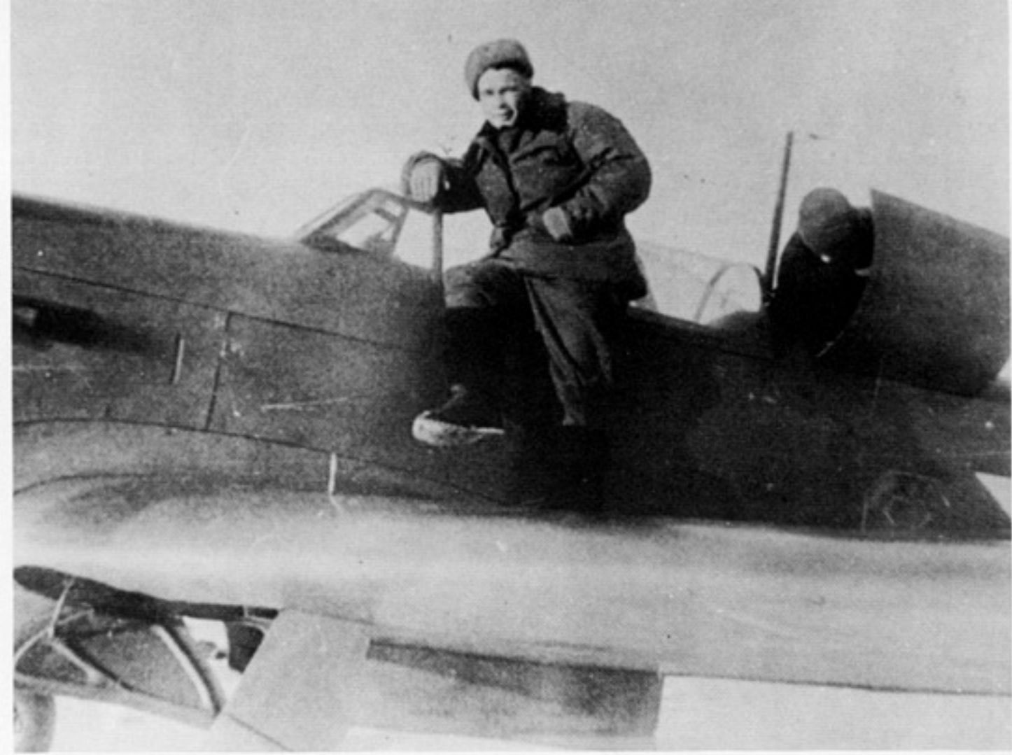
(Above Right) A Soviet pilot poses on his Yak 9. The roomy compartment behind the Cockpit is typical of the 'heavy' fighter series. The Yak 1M and Yak 3 'light' fighters did not have a compartment behind the cockpit. (Musée de l'Air)
