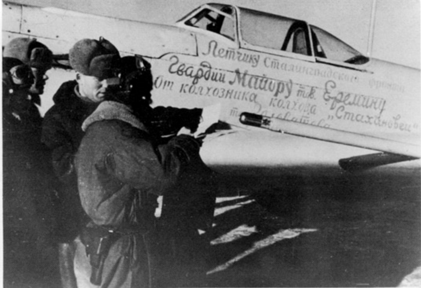
(Above Left) Russian pilots being briefed in front of a White camouflaged Yak 1M donated by Farmers from Stakhanov. The inscription was applied in Red. The pitot tube was mounted on the port wing. The early Yak 1M did not have a jettisonable canopy. (Von Hardesty)
