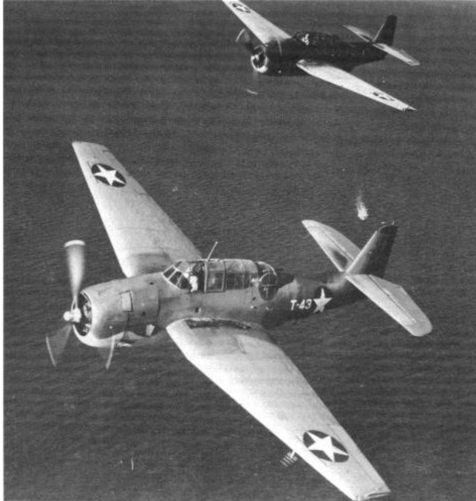
A pair of TBF-1s of an Operational Training Squadron pass over the wake of a submarine's periscope (just behind the tail of the lead Avenger) while conducting anti-submarine training off Florida's east coast during early 1943. The pilots canopy has a slot at the top for the radio antenna mast. (Grumman)
