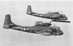
The first production OV-1A (59-2500) and the first production OV-1B (59-2621) in formation over Long Island, New York during 1961. The OV-1B carried an eighteen foot SLAR antenna pod attached to the starboard fuselage side. (Grumman)
