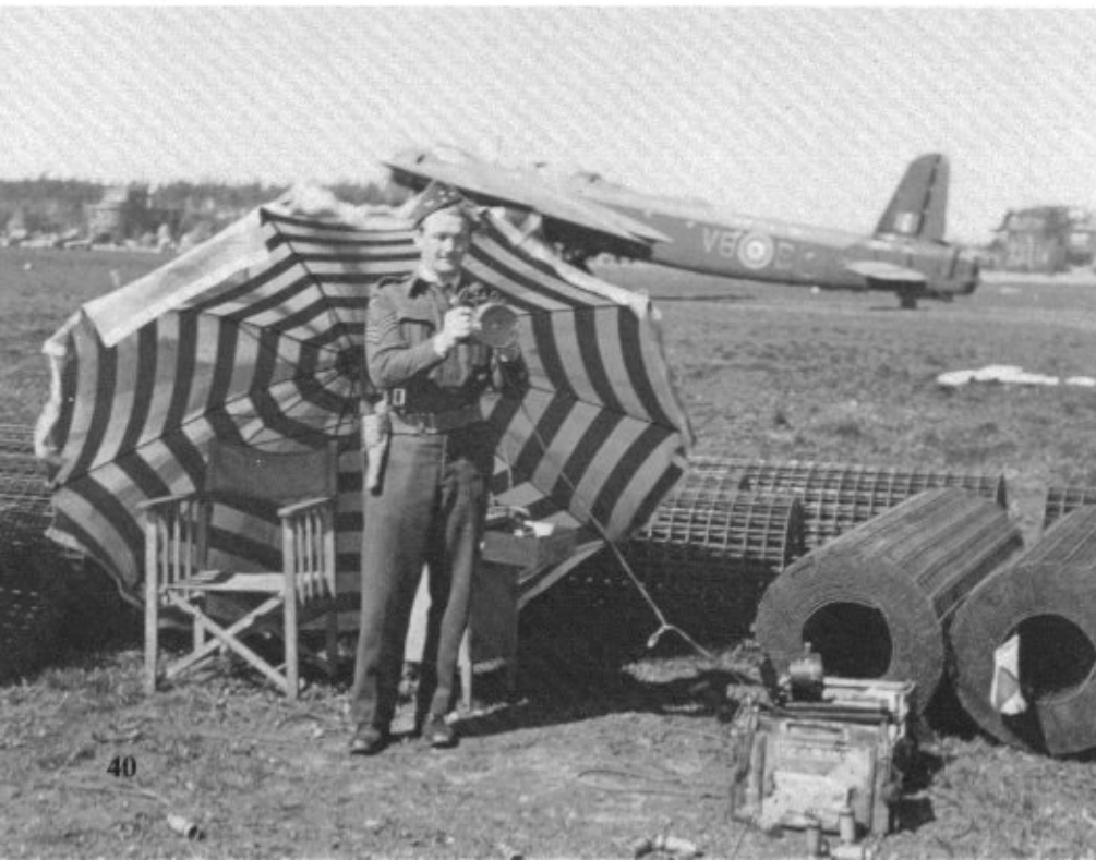
Rolls of Summerfield tracking, used for temporary airfield surfaces, surround this RAF SGT equipped with a signal lamp on an airfield in Europe, as a No 570 Squadron Stirling Mk IV taxis past.
