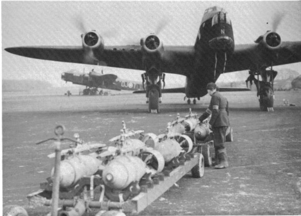
The engines of this Stirling Mk I (N - Nuts) of No 149 Squadron at either Mildenhall or Lakenheath, are run up prior to arming the bomber with its bomb load. The protective covers are still in place on the pitot tube masts. No 149 Squadron was the fourth Bomber Command unit to be equipped with the Stirling.
