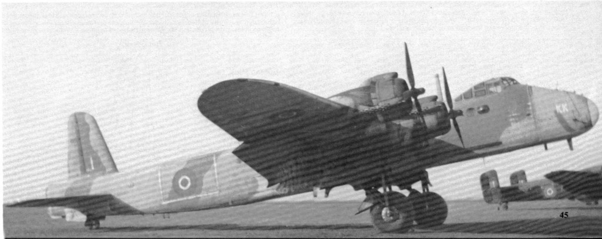
(Above) No 242 Squadron at Stoney Cross was the second Stirling unit convert to the Mk V and this aircraft shows this squadron's method of displaying the squadron and aircraft code letters. The code is carried as small Black letters on each side of the nose. Even though the Mk V was strictly a transport, it retained the bomb bay doors and controls.
