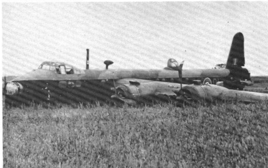
This No 214 (Federated Malay States) Squadron Stirling Mk I Series III rests on her belly after suffering battle damage on the night of 27/28 June 1942. The aircraft is minus the port horizontal stabilizer and is peppered with shell holes from Luftwaffe fighter attacks. The crew, led by Australian pilot SGT Griggs, downed three fighters before staggering home to Stradishall on two engines.
