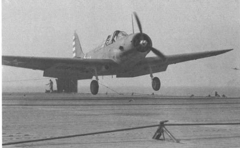
A TBD-1 makes an arrested landing aboard USS LONG ISLAND (AVG-1) during February of 1942. The LONG ISLAND was a motorship that was converted to a training carrier for Advanced Carrier Training Groups (ACTGs). (National Archives)
