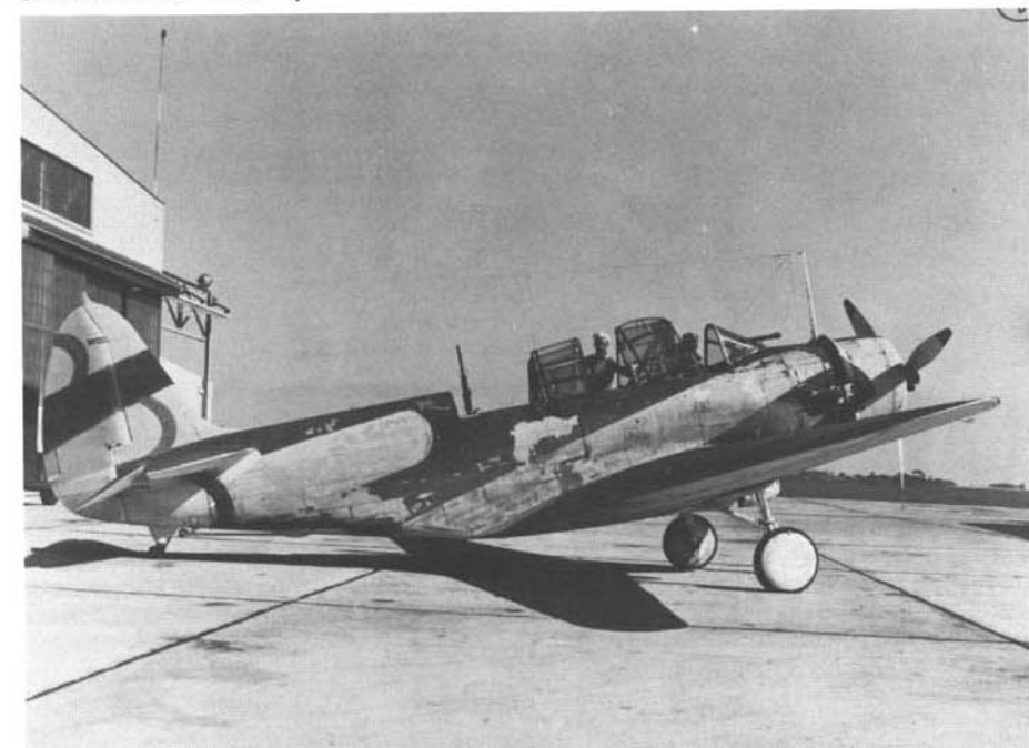
This Devastator (BuNo 0339) of VT-3 assigned to USS SARATOGA carried the Barclay Design 8 pattern. The camouflage paints used were water based and weathered rapidly. (USN/B. Cressman via Jim Mesko)
