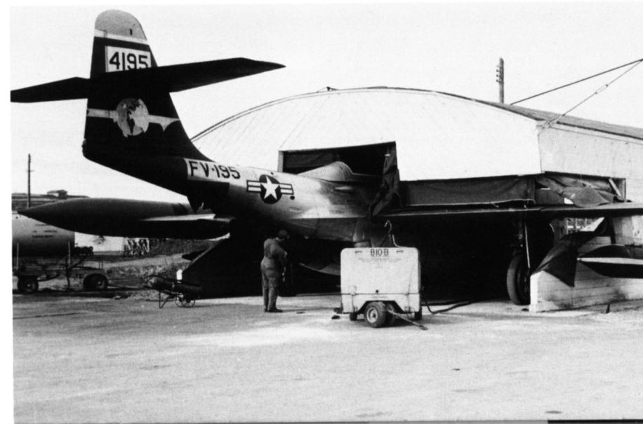
Small sheds were built in cold climates to shield aircraft and maintenance personnel during non-major equipment maintenance. Some of the electronic gear carried on the F-89 was sensitive to cold and had to be kept warm during testing. This shed fits perfectly around a 433rd FIS F-89D at Ladd AFB. (John Finiello)
