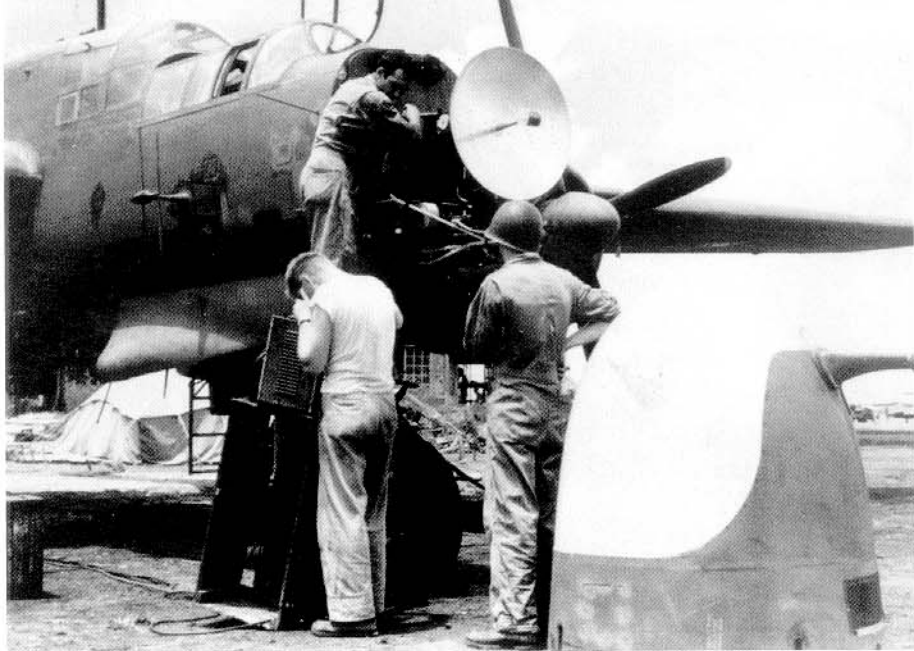
Ground crews perform maintenance on the SCR-720 airborne intercept (AI) radar in the nose of a P-61A on Saipan during July of 1944. The radome was made of fiberglass and left unpainted, giving it a light color. (Dave McLaren)
