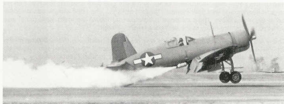
This F4U-1A was the sixth production Corsair. It was modified by Vought to be the first F4U fitted with the enlarged canopy. It greatly increased pilot visibility and soon replaced the birdcage canopy on the production line. (National Archives)
