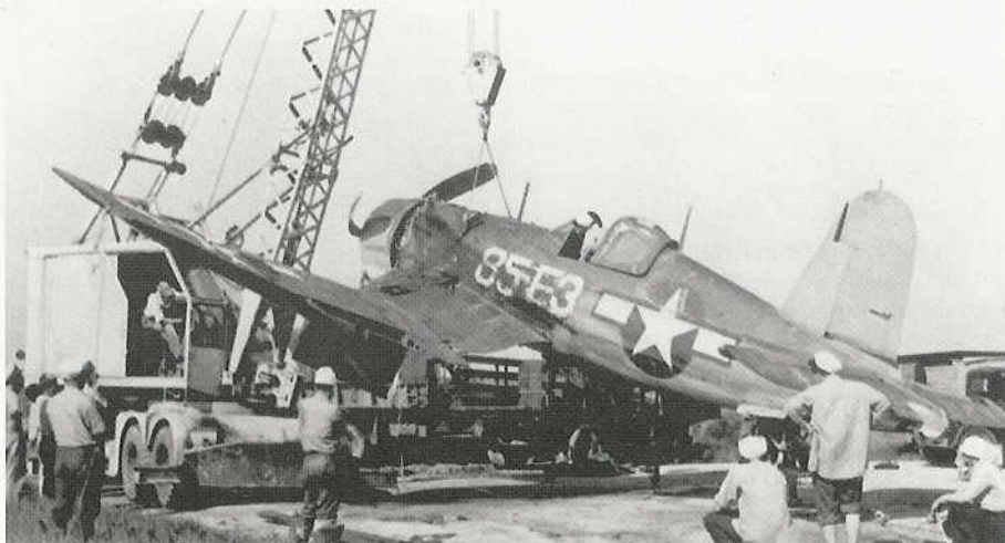
This Goodyear FG-1A (BuNo 14609/KD-178), parked on the Goodyear factory ramp at Akron, Ohio on 8 July 1944, was painted overall Gloss Sea Blue and carried the markings of the British Royal Navy. Royal Navy Corsairs had eight inches clipped off the wingtips to allow the aircraft to fit in the hangar decks of British carriers. (Goodyear via Nick Hauprich)
