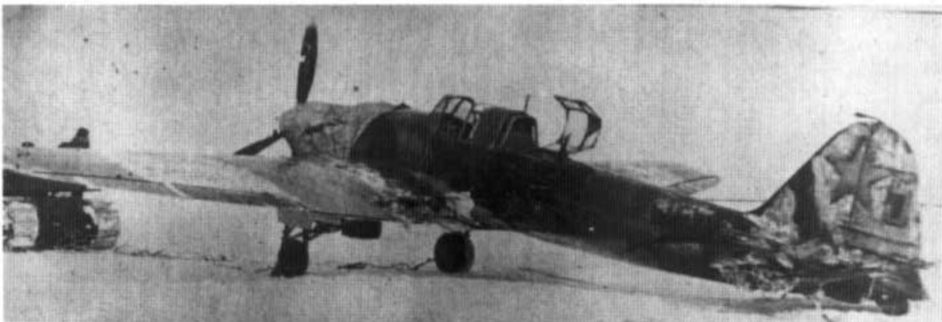
The Stormovik could absorb a lot of battle damage and still bring its crew home. This Il-2M, Yellow 5, has had the port elevator nearly shot away and there is severe damage to the port wing root as well. The aircraft was camouflaged Black-Green and Olive Drab with a Red arrow on the fuselage. (G.F. Petrov)
