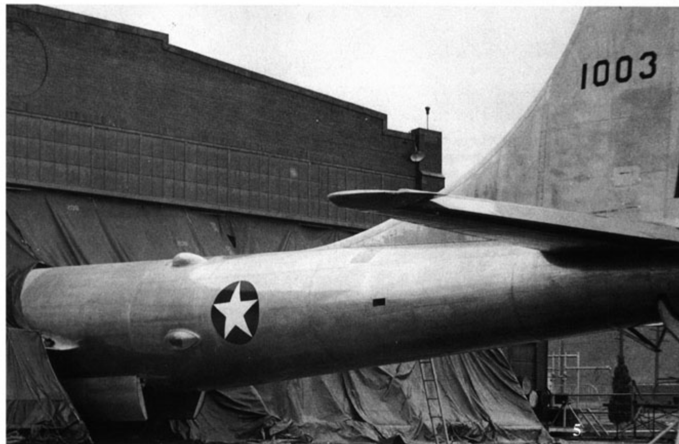
Rollout of the XB-29 came during early September of 1942. The tail bumper, small tail gunners windows, and larger rudder were found only on the XB-29s (Peter Bowers)
