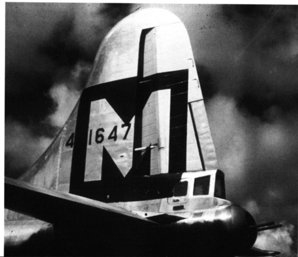
(Below) This 19th BG B-29 carries only the twin .50 caliber machine guns common to 21st Bomber Command aircraft. (Ron Witt)
