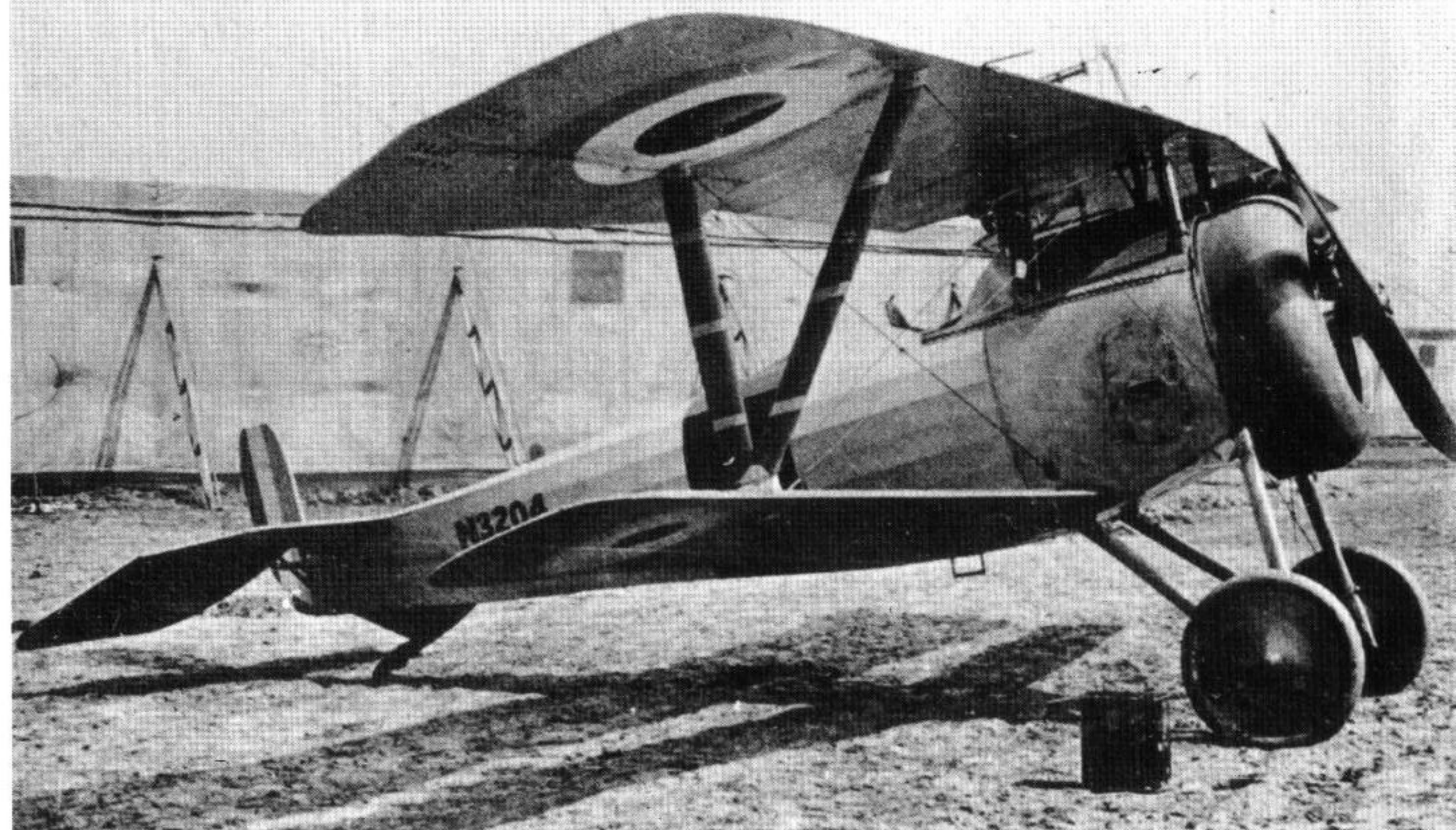
This Nieuport 17bis (N3204) served with No.6 Naval Squadron at La Bellevue about March 1917. Armed with the standard synchronized Vickers gun and powered by a Clerget 9B rotary engine it was lost in combat with Vzfw Riesinger of Jasta 12 on 6 June 1917. The Nieuport's pilot, Flight Lieutenant F.P. Reeves, was killed.
