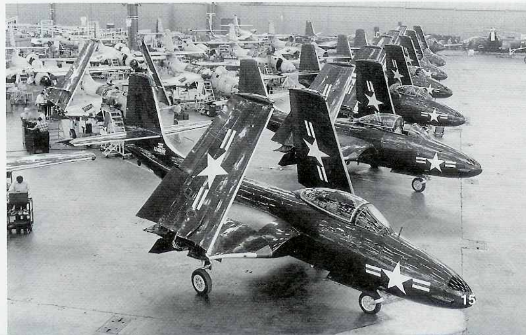
Eight brand new F2H-2s await installation of their wingtip tanks at McDonnell's St. Louis factory. Ten other Banshees in various stages of construction follow on the assembly area. McDonnell built 406 F2H-2s for the Navy and Marines, making this the most prolific Banshee variant. (MDC)
