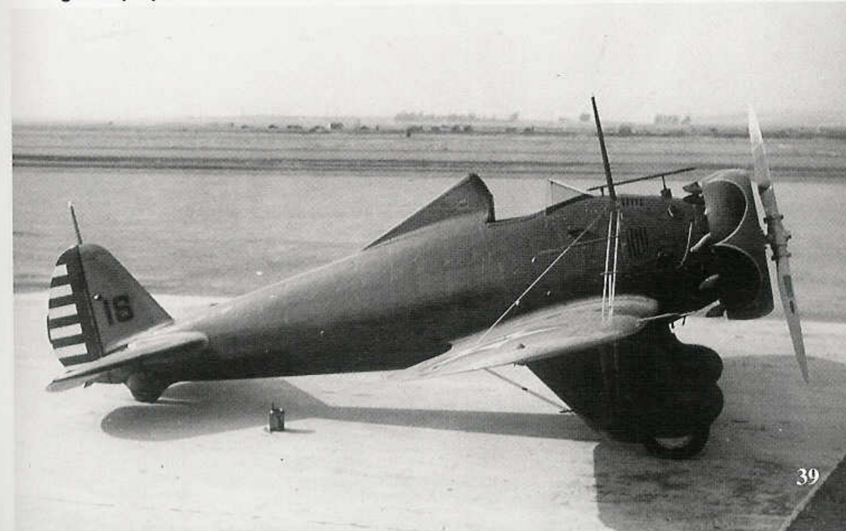
This pair of P-26As of the 77th Pursuit Squadron, 20th Pursuit Group at Barksdale Field, LA during 1934 carry the early style of 20th PG cowl ring markings. The cowl ring had a Red scallop with White trim and the engine facing was also painted Red. The long tube extending from in front of the windscreen was the telescopic gun sight. All P-26 variants were armed with a pair of .30 caliber machine guns mounted in the lower fuselage and firing through the propeller arc. Robert Esposito)
