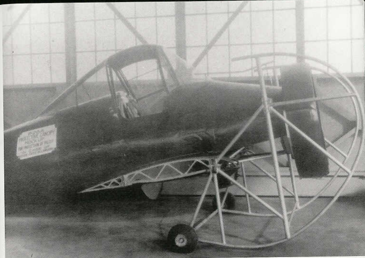
The problem of P-26 turnovers was so great that Boeing engineers came up with this very novel P-26 protective cockpit mockup during 1936. Although it would have protected the pilot in the event of a noseover/turnover accident, the drag was too great and this cockpit was not adopted. (AFM)
