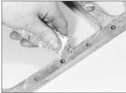
13.11a Where a sump spacer plate is fitted, apply a coat of suitable sealant to the plate upper surface . . .
