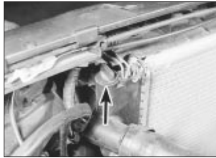
20.4c Radiator bleed screw (arrowed)
