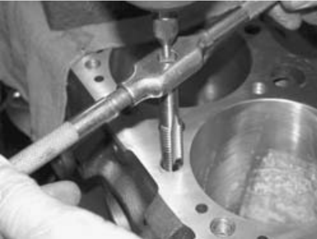
FIGURE 3-31 Use a special tap for the insert.
