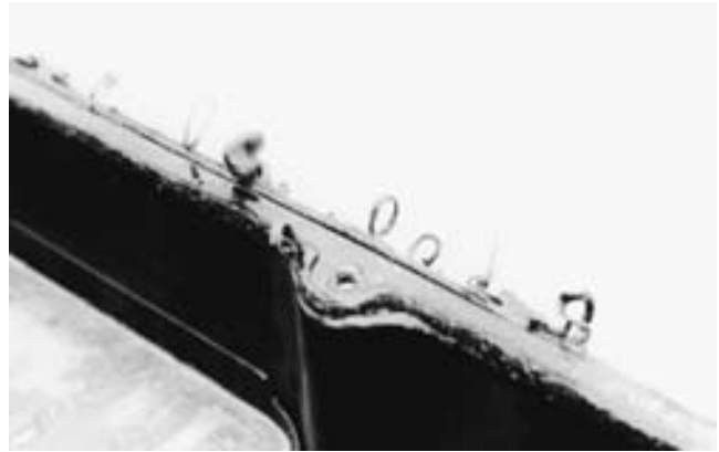
FIGURE 30-51 Improperly sealed valve cover gasket. Note the use of RTV silicone sealant on a cork-rubber gasket. The cover bolts were also overtightened, which deformed the metal cover around the bolt holes.
