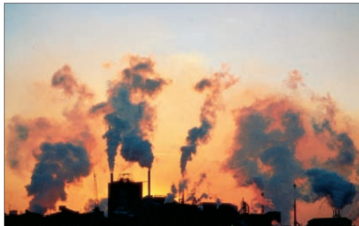
Figure 2.13 Emissions of sulfur dioxide from a coal-burning power plant. Airborne pollutants such as sulfur dioxide dissolve in water vapor to form acidic solutions. They are a component of acid rain.
