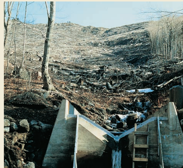
Figure a Weir used to measure the volume and nutrient content of water leaving a watershed by streamflow.
