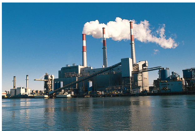
FIG. 5.9 Water is a product of the combustion of hydrocarbons. Here we see clouds of condensed water vapor coming from the stacks of an oil-fired electric generating plant during the winter. (Sandra Baker/Liaison Agency, Inc./Getty Images.)
