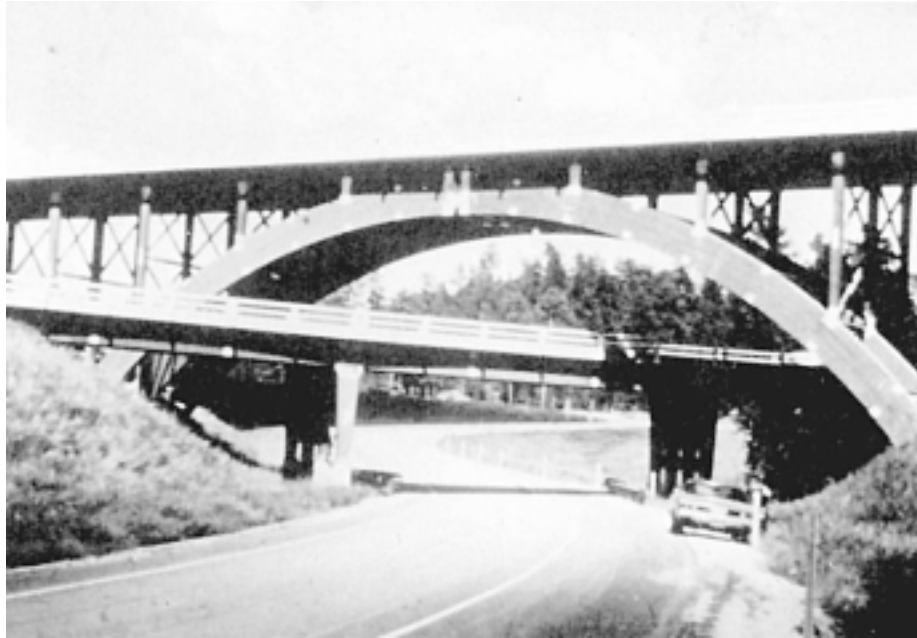
Figure 11-31 Highway bridges supported by glued laminated timber beams. (Courtesy of American Institute of Timber Construction)
