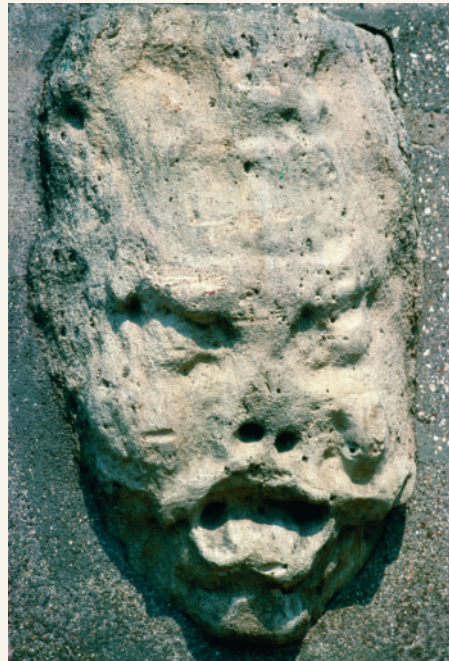
FIGURE 6.B Acid rain accelerates the chemical weathering of stone monuments and structures. (Photo by Adam Hart-Davis/Science Photo Library/Photo Researchers, Inc.)
