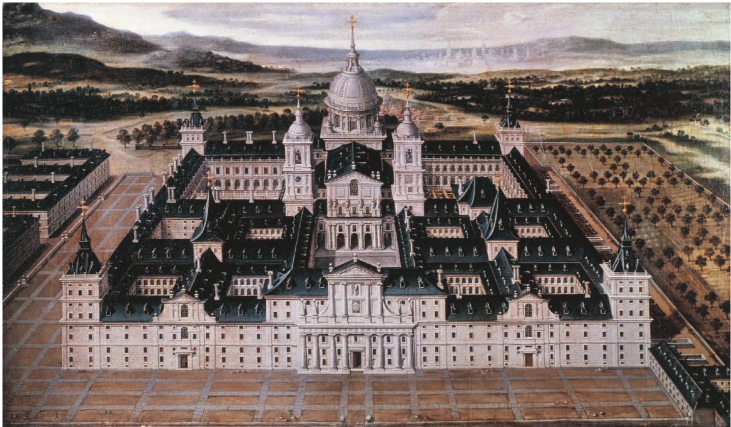
23-24 JUAN DE HERRERA and JUAN BAUTISTA DE TOLEDO, El Escorial, near Madrid, Spain, 1563–1584 (detail of an anonymous 18th-century painting).
