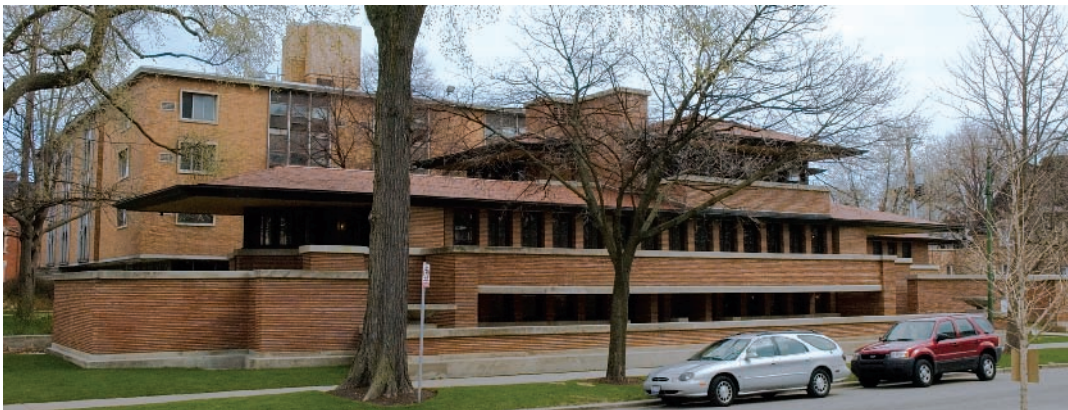
35-77 FRANK LLOYD WRIGHT, Robie House, Chicago, Illinois, 1907–1909.
