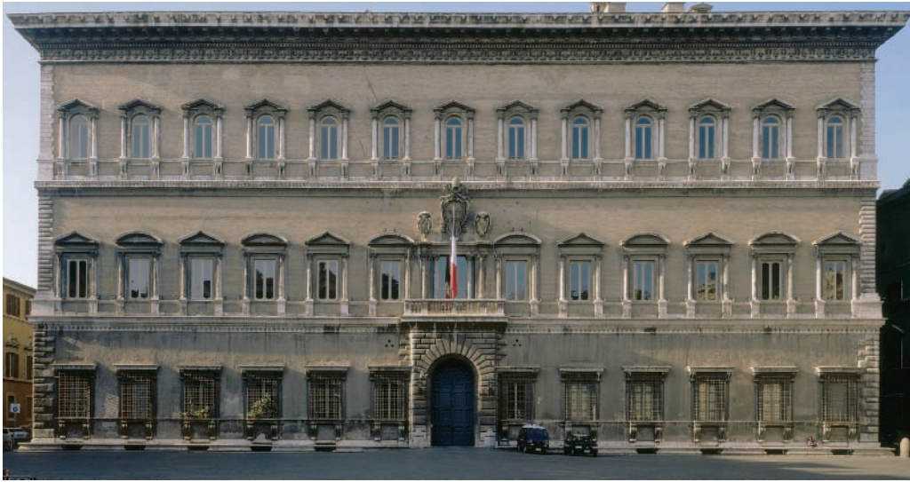
22-27 ANTONIO DA SANGALLO THE YOUNGER, Palazzo Farnese (looking southeast), Rome, Italy, 1517–1546; completed by MICHELANGELO BUONARROTI, 1546–1550.
