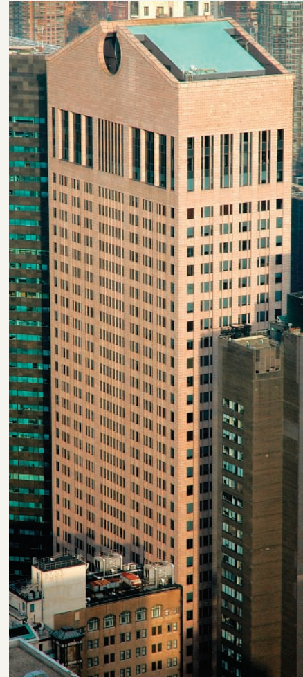
36-64 PHILIP JOHNSON and JOHN BURGEE (with SIMMONS ARCHITECTS), AT&T (now Sony) Building, New York, 1978–1984.
