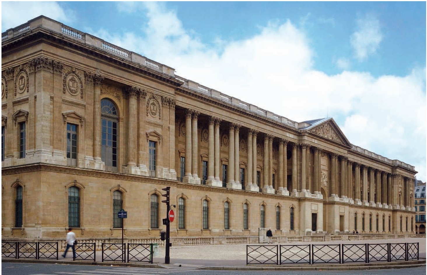
25-31 CLAUDE PERRAULT, LOUIS LE VAU, and CHARLES LE BRUN, east facade of the Louvre, Paris, France, 1667–1670.
