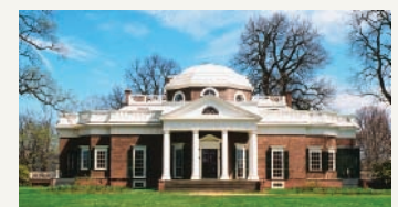
Jefferson, Monticello , Charlottesville, 1770-1806
