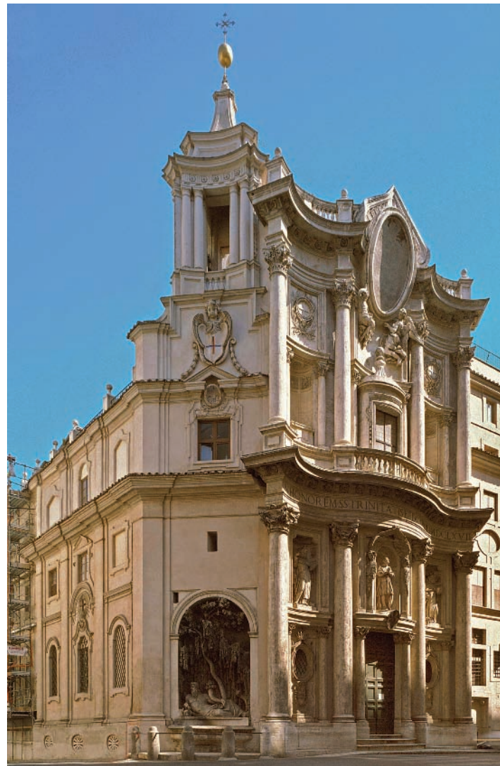
24-9 FRANCESCO BORROMINI, facade of San Carlo alle Quattro Fontane, Rome, Italy, 1665–1667.
