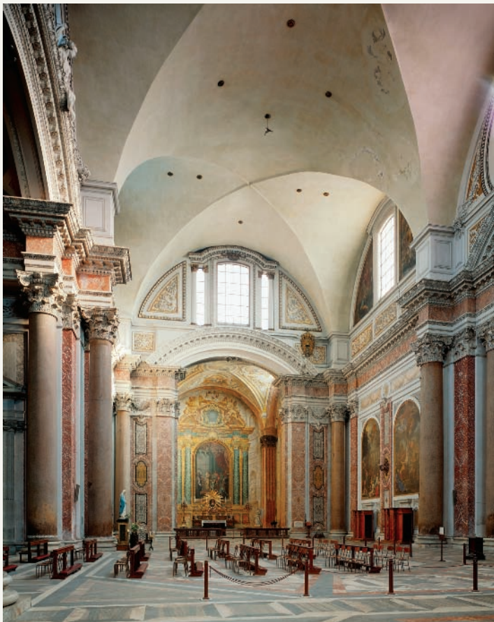
Roman hall with groin vaults (Baths of Diocletian [Santa Maria degli Angeli], Rome, Italy, ca. 298–306)
