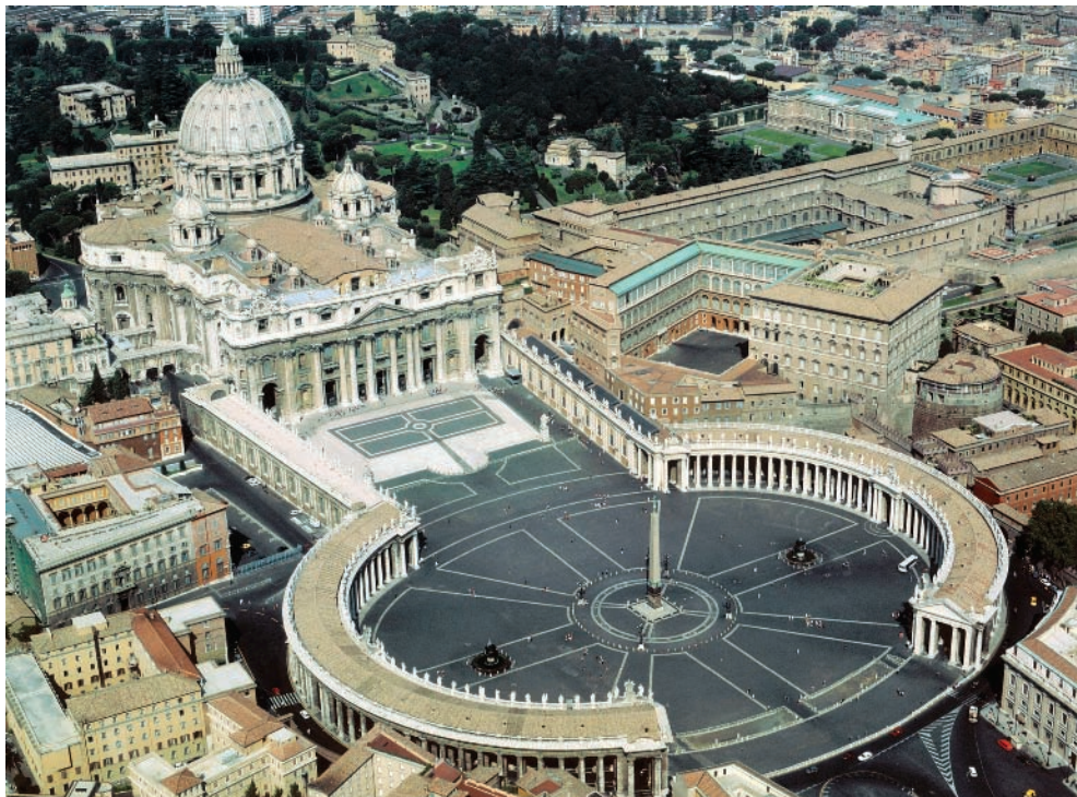
24-4 Aerial view of Saint Peter's, Vatican City, Rome, Italy. Piazza designed by GIANLORENZO BERNINI, 1656–1667.
