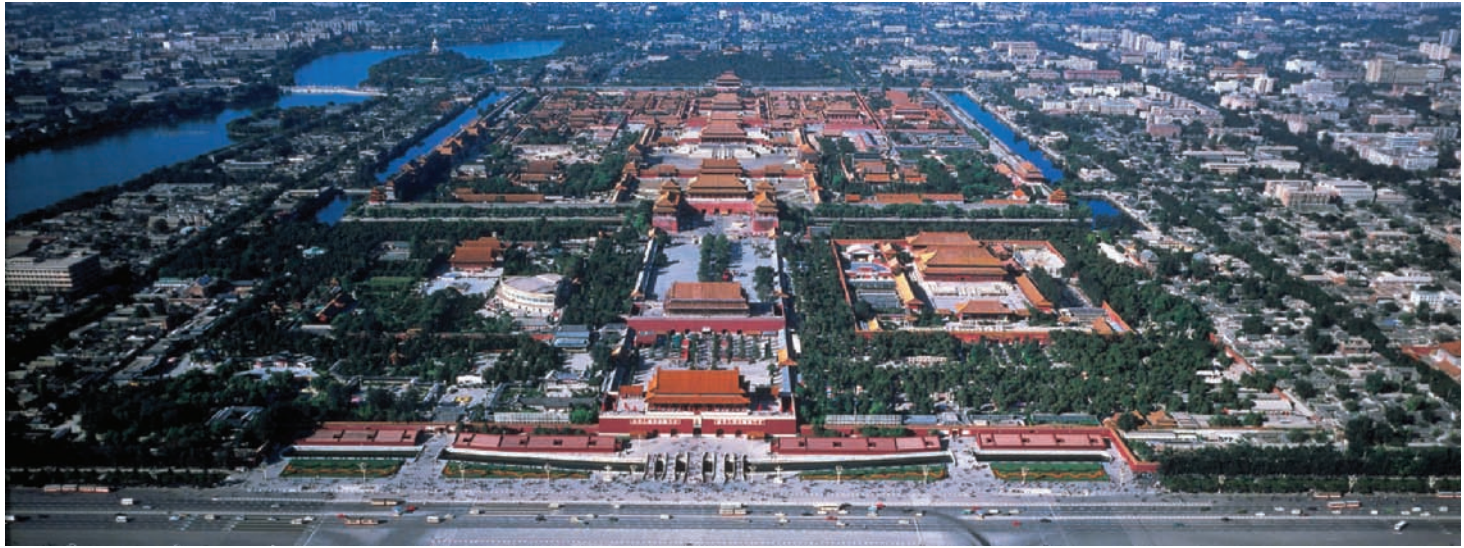
27-6 Aerial view (looking north) of the Forbidden City, Beijing, China, Ming dynasty, 15th century and later.
