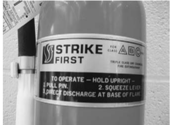
FIGURE 1-43 A typical fire extinguisher designed to be used on class A, B, or C fires. (Courtesy of James Halderman)
