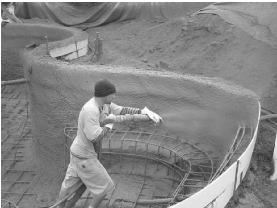
FIGURE 7.40 Constructing a swimming pool using shotcrete.
