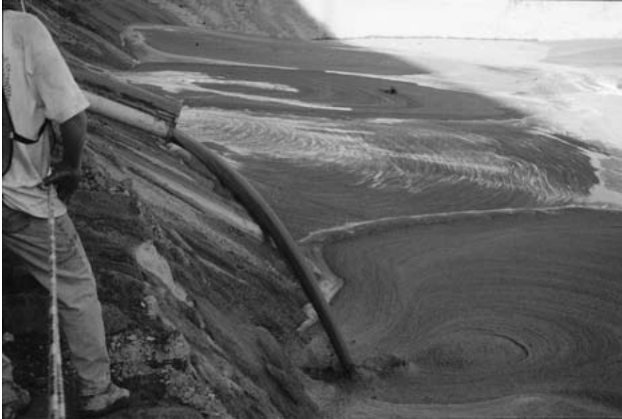
FIGURE 7.39 Filling a sink hole with flowable fill.
