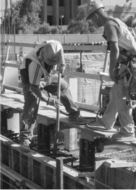
FIGURE 7.11 Consolidating concrete with an internal vibrator.
