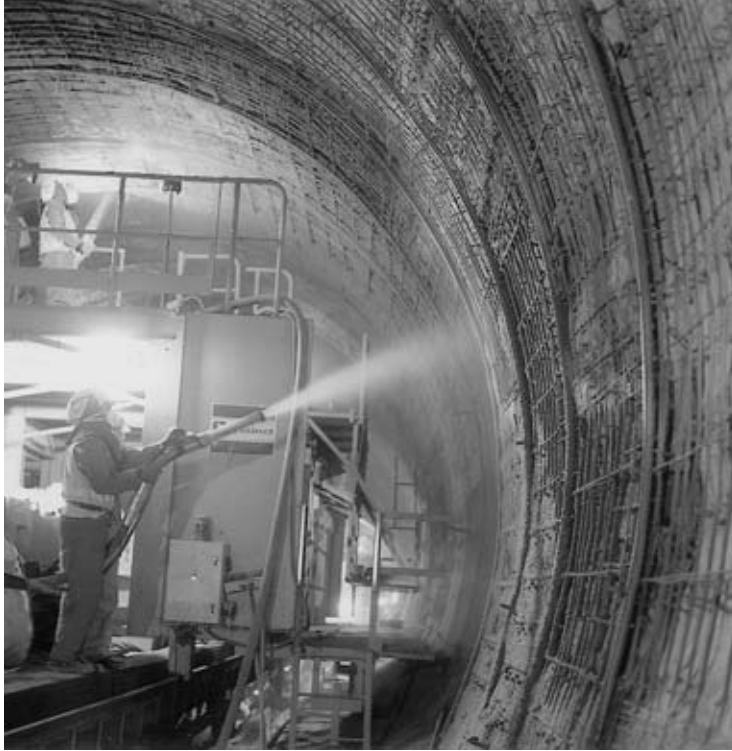
FIGURE 7.41 Shotcrete used in lining a tunnel.
