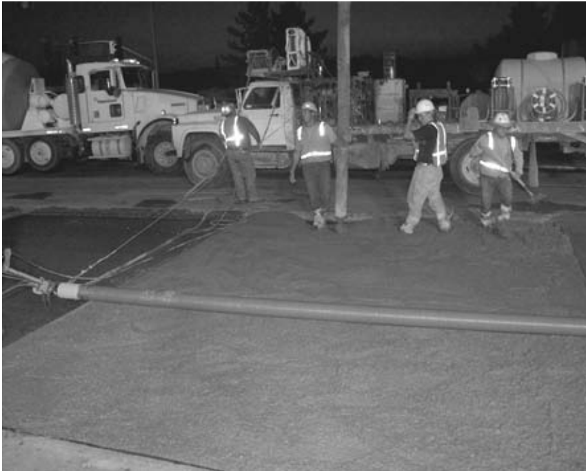
FIGURE 7.15 Spreading concrete with a straightedge.
