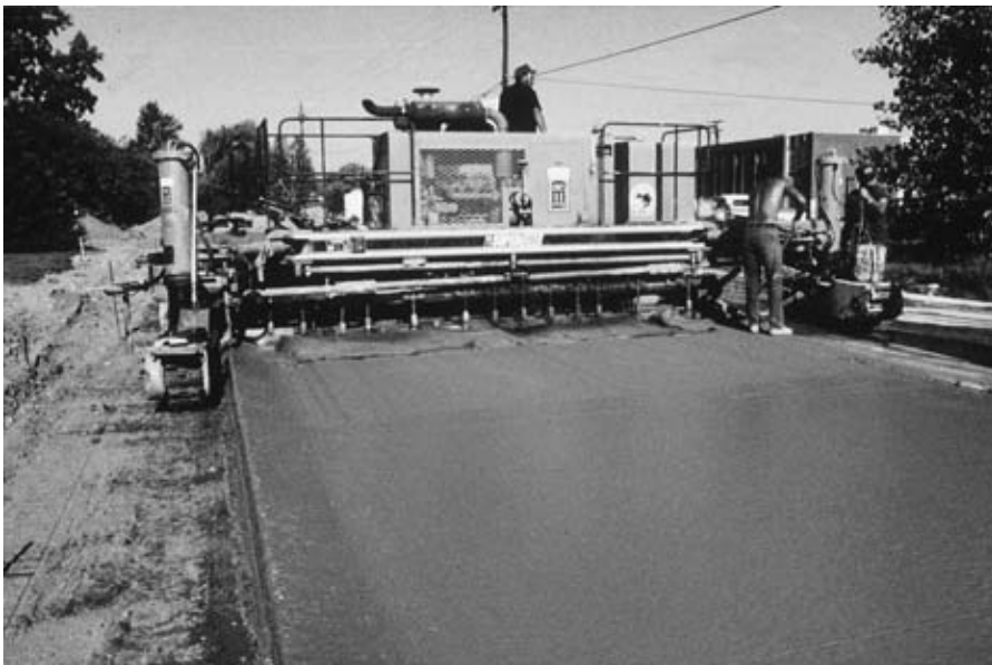
FIGURE 7.8 Placing concrete pavement with a slip-form paver.
