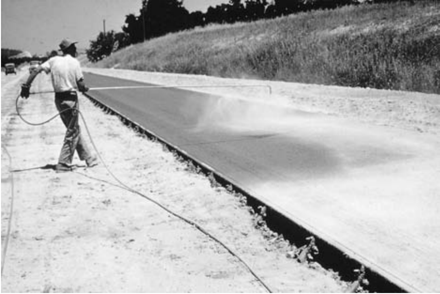
FIGURE 7.25 Curing concrete by manually applying membrane forming compound.
