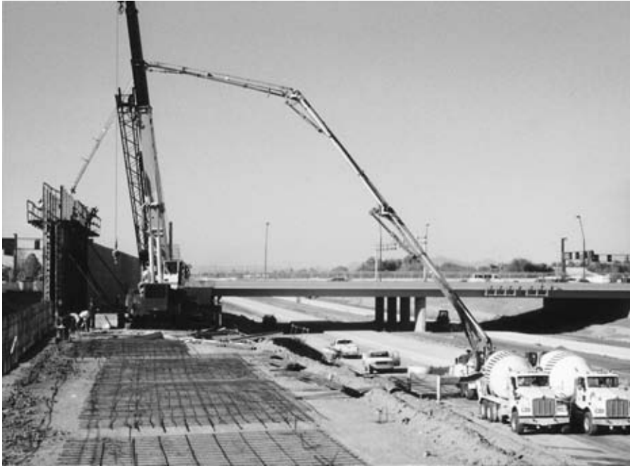
FIGURE 7.10 Pumping concrete in a retaining wall.
