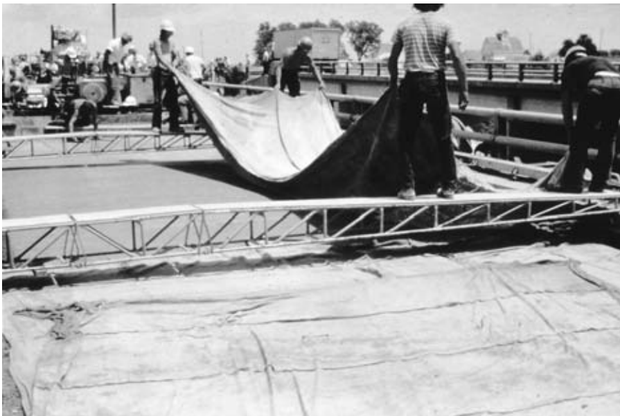
FIGURE 7.23 Curing concrete with impervious fabrics.
