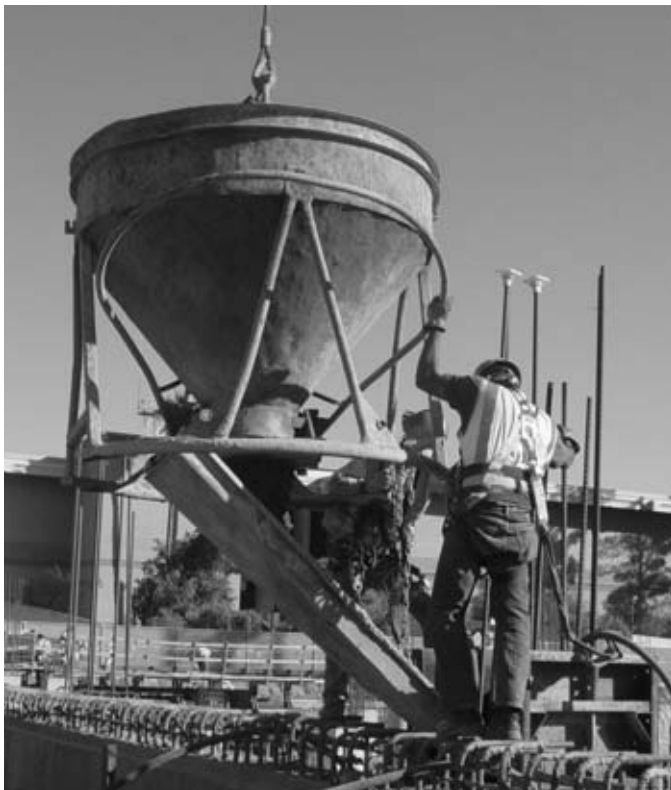
FIGURE 7.9 Depositing concrete using a 2-1/2 cubic yard bucket.
