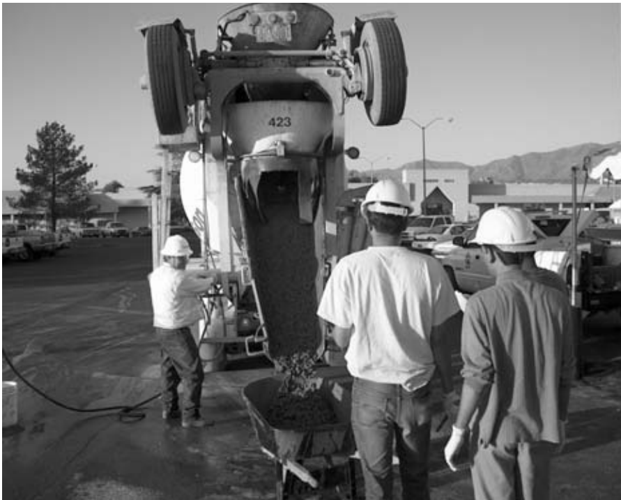
FIGURE 7.6 Loading concrete in a wheelbarrow.
