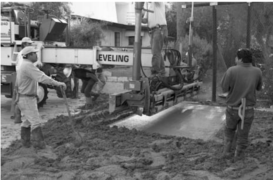
FIGURE 7.18 Finishing concrete with a laser level.
