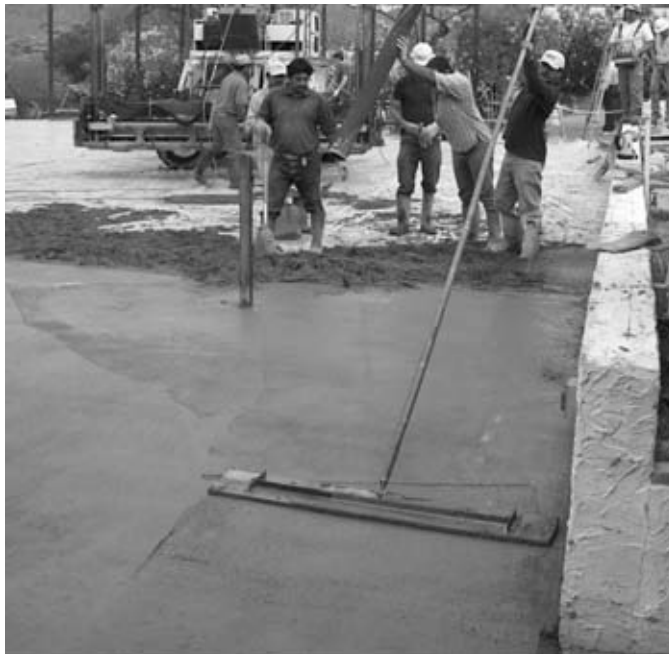
FIGURE 7.16 Finishing concrete with a straightedge.
