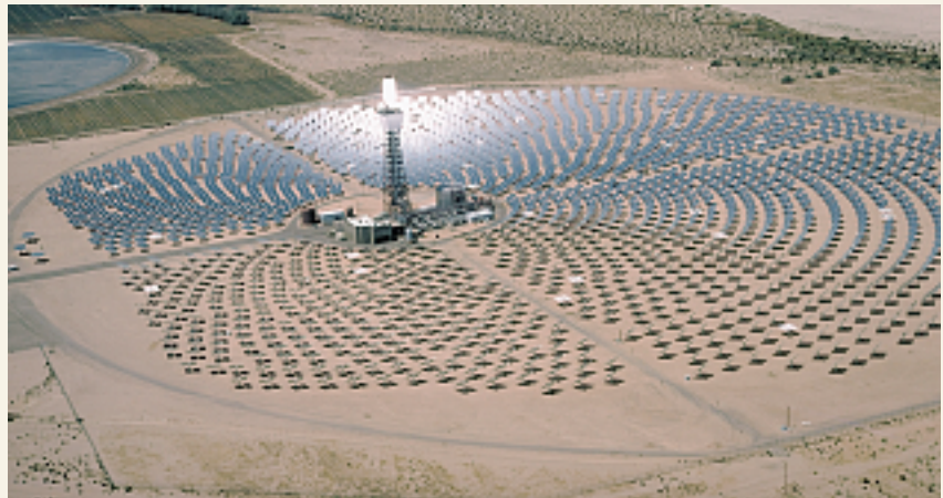
FIGURE 2-F Solar One, a solar installation used to generate electricity in the Mojave Desert near Barstow, California. (Photo by Thomas Braise/Corbis/Stock Market)
