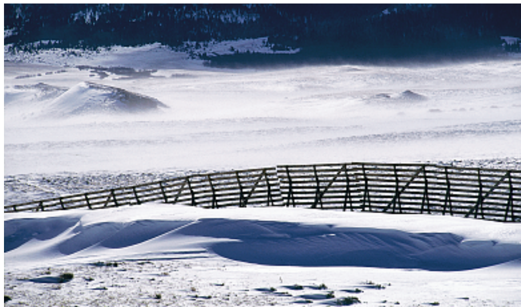
FIGURE 6-18 A snow fence slows the wind, thereby decreasing the wind's ability to transport snow. As a result, snow accumulates on the downwind side of the fence. (Photo by Stephen Trimble)
