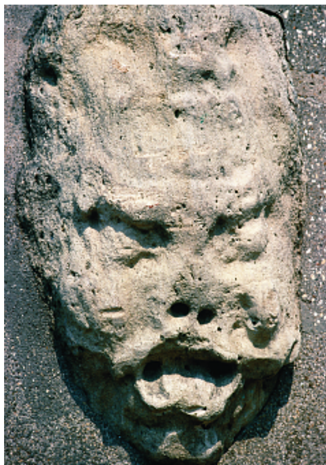
FIGURE 13-19 Acid rain accelerates the chemical weathering of stone monuments and structures. (Photo by Adam Hart-Davis/Science Photo Library/Photo Researchers, Inc.)
