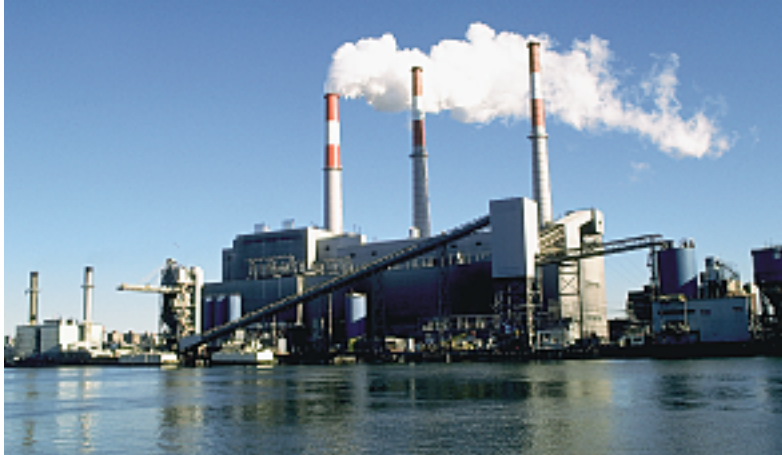
FIGURE 13-17 Tall stacks improve local air quality by releasing pollutants at greater heights where winds are stronger. However, such stacks promote the long-distance transport of pollutants that may ultimately contribute to acid precipitation far from their source. (Photo by Sandra Baker/Liaison Agency, Inc.)
