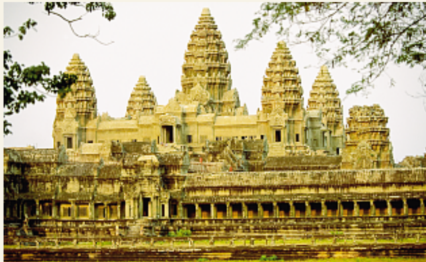
FIGURE 15-C This ancient temple at Angkor Wat, Cambodia, was built of bricks made of laterite. (Photo by R. Ian Lloyd/Corbis/Stock Market)
