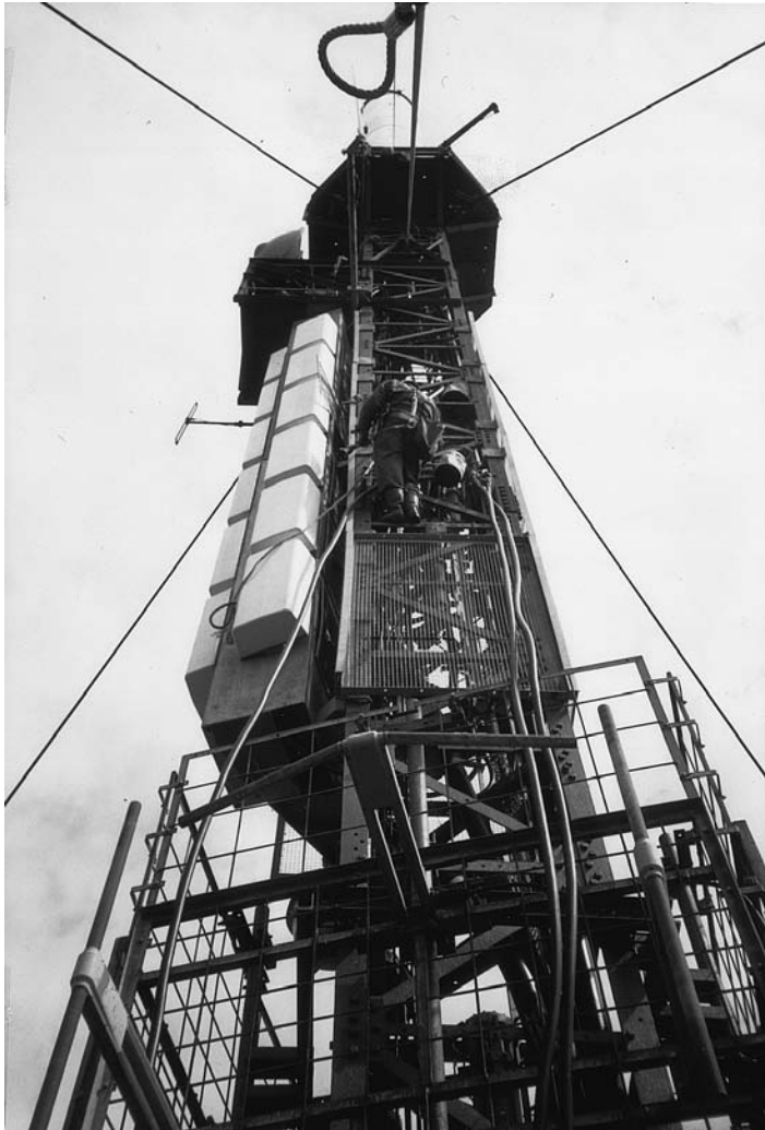
Figure 2.11 BBC mast Isle of Wight (Courtesy Crown Castle International)
