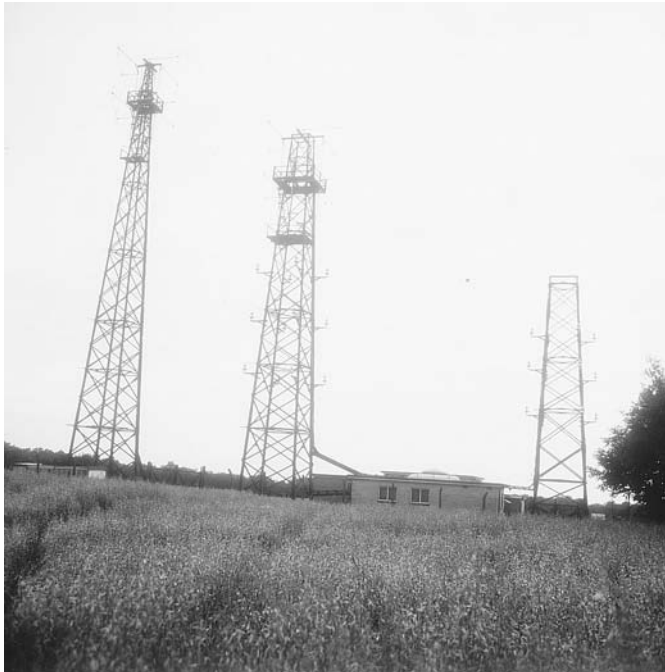
Figure 2.14 ATC UHF and VHF antenna installation (Courtesy NATS)
