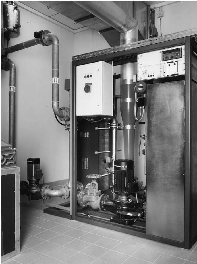
Figure 2.3 Telefunken dummy load (Courtesy Telefunken Sendertechnik GmbH)
