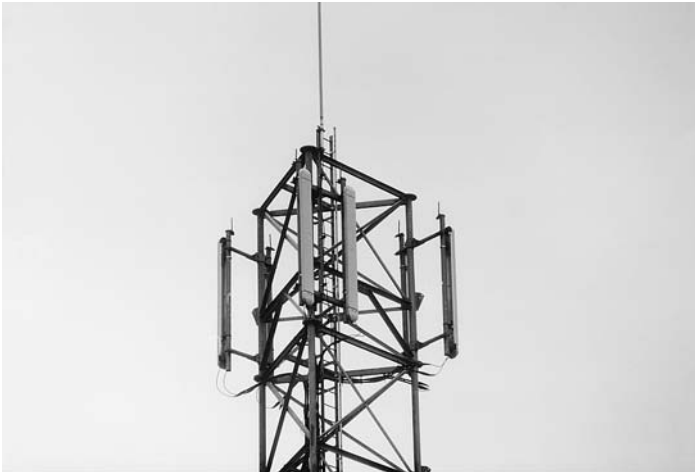
Figure 6.22 Tower with inside ladder (Courtesy of E. Randall)
