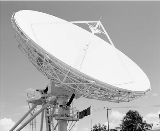
Figure 2.15 Satellite ground station (Courtesy Cable and Wireless)
