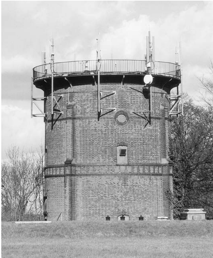
Figure 6.21 Roof mounted equipment – round brick tower (Courtesy of E. Randall)
