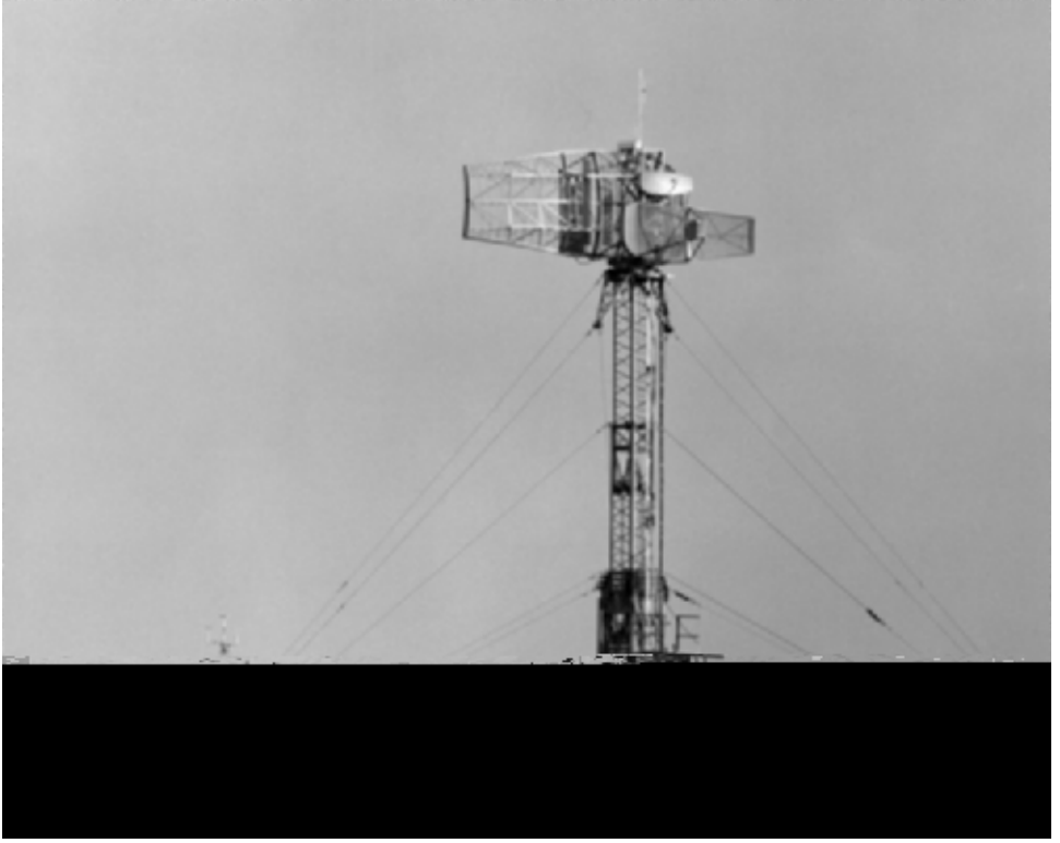
FIGURE 3.1 Phase One equipment at Lethbridge West, Alberta. Antenna tower erected to 60 ft.
