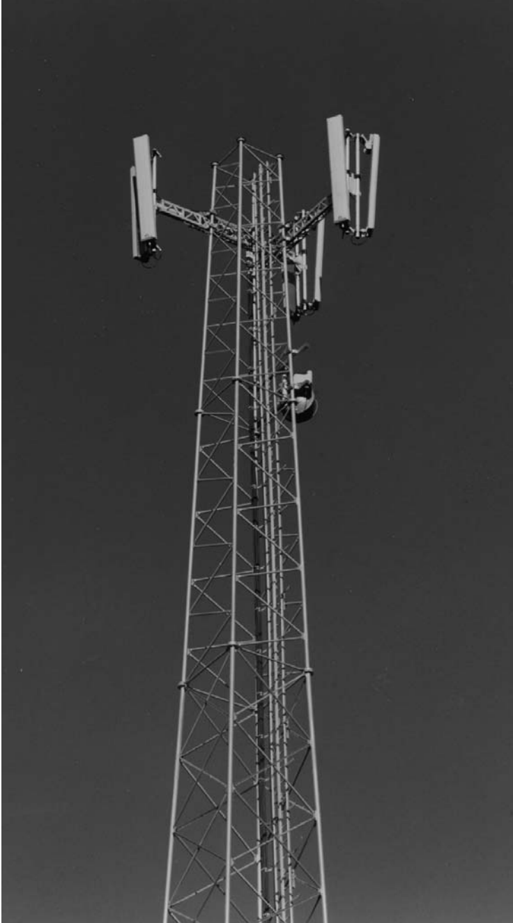
Figure 2.12 Cell site for cellular system.
