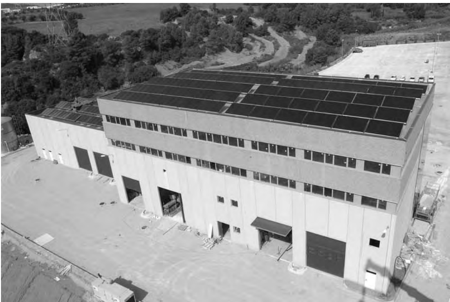
FIGURE 20.40 Parking service Castellbisbal SA, container washing, Spain. Installed capacity: 357 kW th . (From Aiguasol Engineering, Spain. With permission.)
