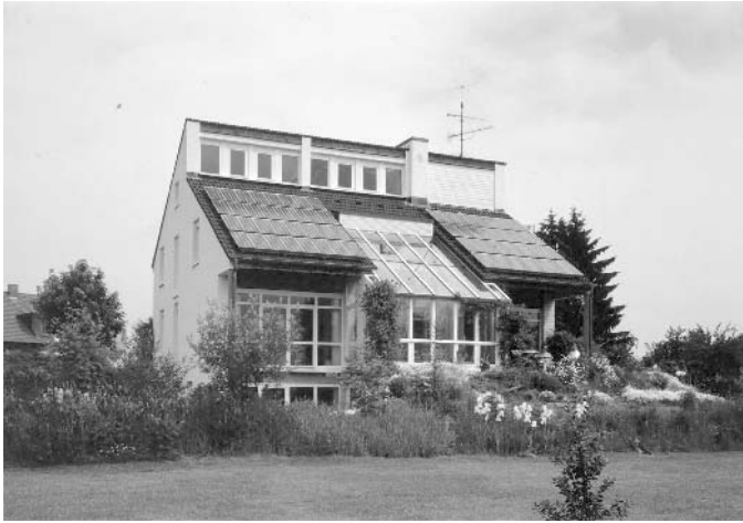
Figure 2.7 Distributed power generation by means of photovoltaics. The roof-integrated photovoltaic system has a peak power of 5 kW
