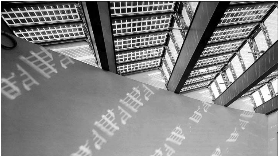
Figure 2.8 Photovoltaic integration into the glazing of a shed roof. In this case, photovoltaic cells serve also as optical shading elements for the space below, preventing overheating under summer conditions
