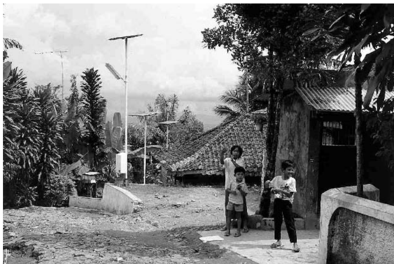
Figure 17.7 Sukatani, the first SHS pilot village in Indonesia, was the origin of the currently running rural electrification programme to electrify one million rural households in Indonesia (Source: Fraunhofer ISE, Freiburg)
