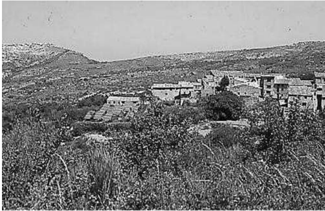
Figure 17.15 PV-Diesel-Hybrid system in Llavería (Source: TTA, Barcelona)
