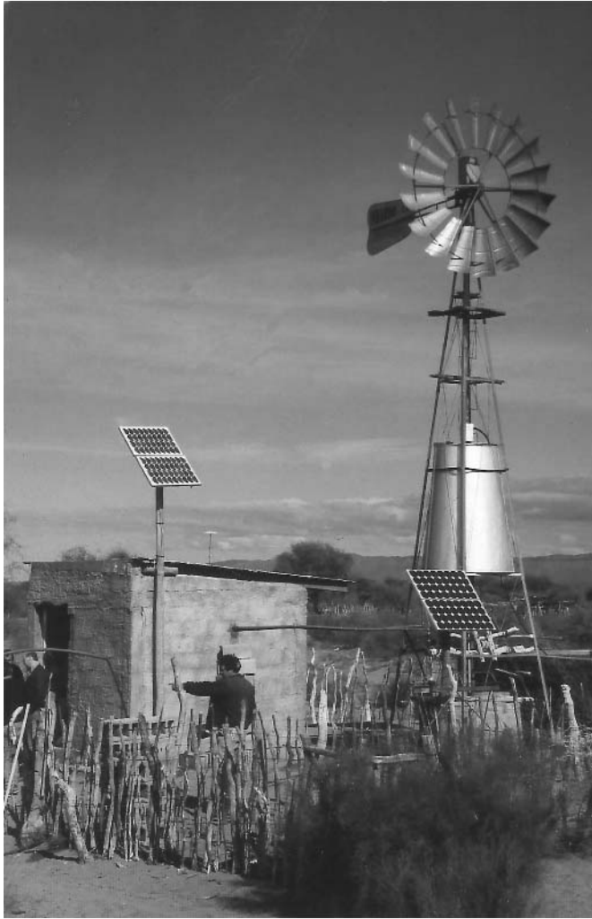
Figure 17.17 Photovoltaically powered purification unit at a wind powered water pump in Balde del Sur de Chucuma/Argentina ( Source: Fraunhofer ISE, Freiburg)
