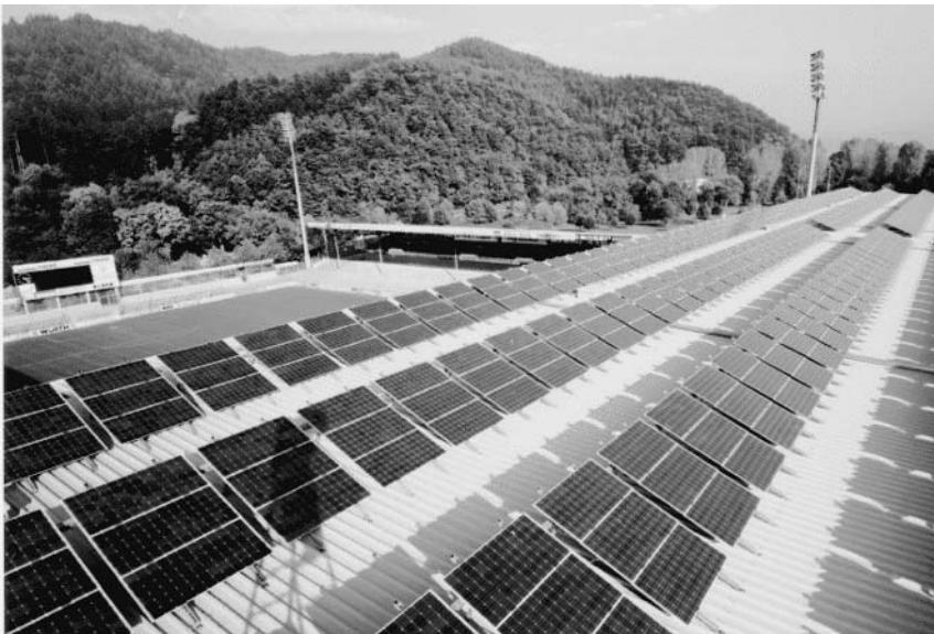
Figure 17.30 Joint ownership PV installation of 100 kW on the soccer stadium Freiburg, Germany [27]
