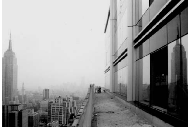
Figure 22.2 Integrated façade system with 14 kWp amorphous silicon modules made by Energy Photovoltaics (EPV) in New Jersey, USA on top of a skyscraper at Four Times Square, New York, USA. The PV modules are the dark regions on the facade near the top. Reproduced from Kiss G, Proc. 2 nd WC Photovoltaic Solar Energy Conversion, 2452–2455 (1998) with permission by Gregory Kiss [7]
