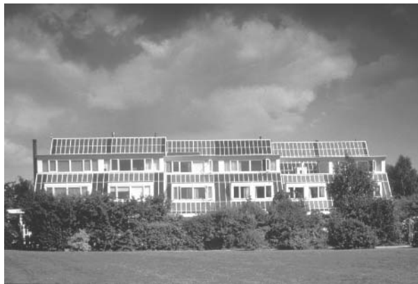
Figure 22.3 Roof integration in a renovation project with the Shell Solar/BOAL profiles in Leiden (NL), providing a 2.1 kWp system per house. The PV roof is an impermeable layer. Reproduced from Maycock P et al. , Building with Photovoltaics , 78–81, Ten Hagen & Stam, Den Haag (1995) with permission by NOVEM, R Schropp [10]
