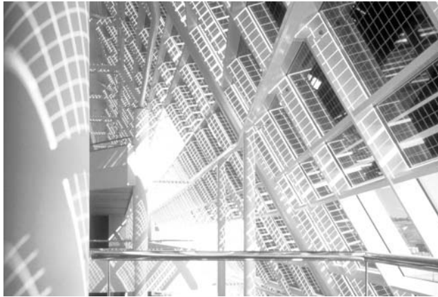
Figure 22.4 Solar office in Doxford Sunderland (UK) with a transparent double-glazing PV system integrated in the façade. The 73 kWp PV system is manufactured by Saint Gobain and mounted in Schüco window frames. Reproduced with permission by Dennis Gilbert
