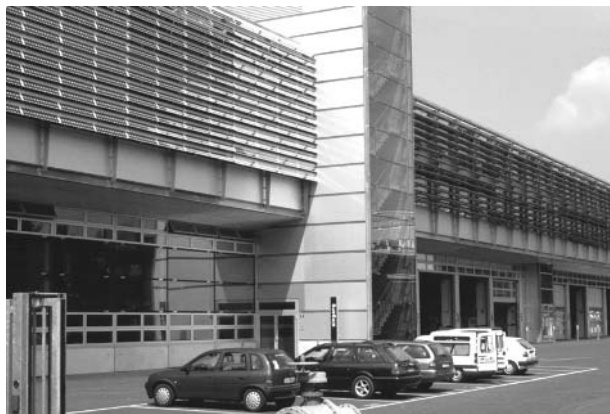
Figure 22.9 Colt shading system that is optimized for sun control. The distance between the louvers with PV modules cause shading on 50% of the PV cells; 47 kWp PV system at Stadtwerke in Winterthur (CH). Reproduced with permission by BEAR Architekten T. Reijenga
