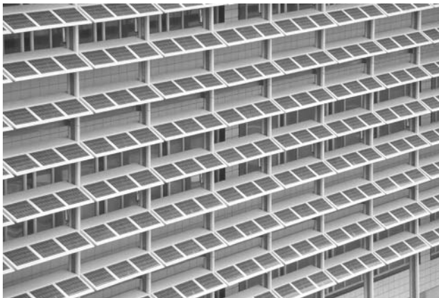
Figure 22.11 South façade of ECN Building 31 in Petten (NL). The shading structure supports the 35 kWp Shell Solar modules. Reproduced with permission by BEAR Architecten T. Reijenga
