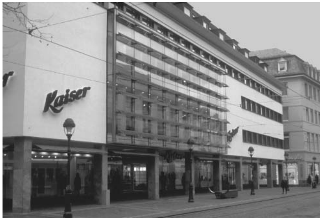
Figure 22.10 Daylight control at the Kaiser fashion house in Freiburg (D). This 4 kWp PV system on louvers is mounted in front of the glass façade and prevents glare inside. The PV louvers are in the center of the figure. Reproduced with permission by BEAR Architecten T. Reijenga
