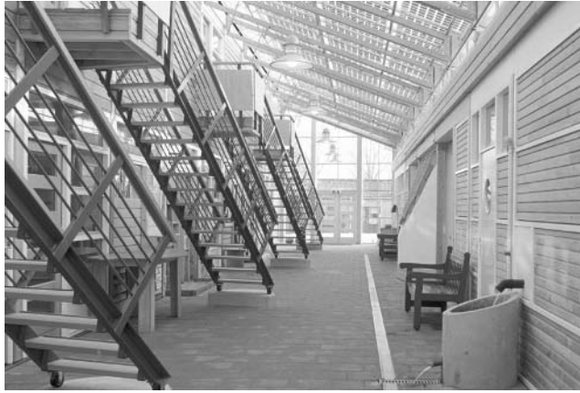
Figure 22.14 Corridor in the Centre for Sustainability De Kleine Aarde in Boxtel (NL). The space is unheated and naturally ventilated. The 6.7 kWp PV system with transparent modules has a double function and reduces the heat load by around 70%. Reproduced from Reijnga T, Böttger W, Proc. 2 nd WC Photovoltaic Solar Energy Conversion , 2748–2751 (1998) with permission by NOVEM, R Schropp [11]
