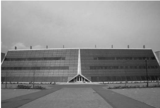
Figure 22.18 The Schüco façade in the Solar office in Doxford, Sunderland (UK) is well engineered. Reproduced with permission by BEAR Architecten T. Reijenga
