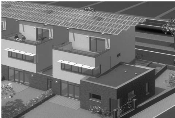
Figure 22.28 This zero-energy project in Etten-Leur (NL) combines different sustainable energy techniques. Each house has a roof structure with 6.2 kWp BP Solar PV modules. The aesthetic integration of the PV system is a completely new concept in housing. Reproduced from Reijenga T, “Energy-Efficient And Zero-Energy Building in the Netherlands”, Proc. International Workshop on Energy Efficiency in Buildings in China for the 21 st Century , CBEEA (Beijing, December 2000) with permission by BEAR Architecten M. van de Laan [30]
