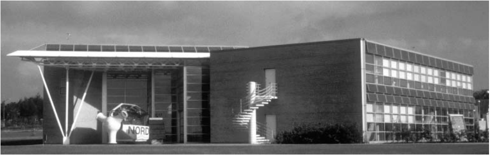
Figure 22.29 Overview of the Brundtland Centre in Toftlund (DK). The glass roof on top of the atrium in the middle of the building has a saw-tooth roof with integrated 9.8 kWp transparent PV modules. Reproduced with permission by BEAR Architecten T. Reijenga
