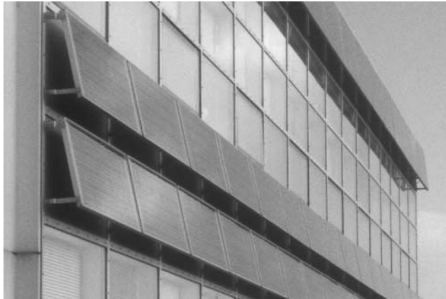
Figure 22.30 PV modules above the windows on the southeast facade. A total of 6 kWp is integrated in the facade. Reproduced with permission by BEAR Architecten T. Reijenga
