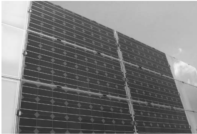
Figure 22.40 BP Solface vertical wall system at the Demosite in Lausanne (CH). Reproduced with permission by EPFL-LESO-PB
