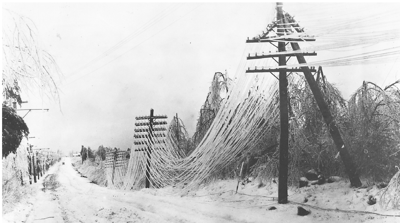
FIGURE 5.28 A heavy coating of freezing rain during this ice storm caused tree limbs to break and power lines to sag.
